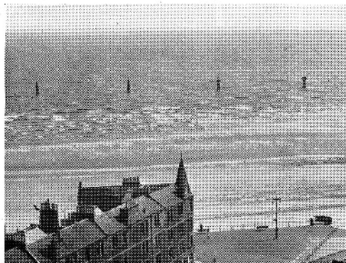
A view of the three intake pipes from the Firth of Forth for cooling purposes. The fourth and right-hand is the return pipe.
